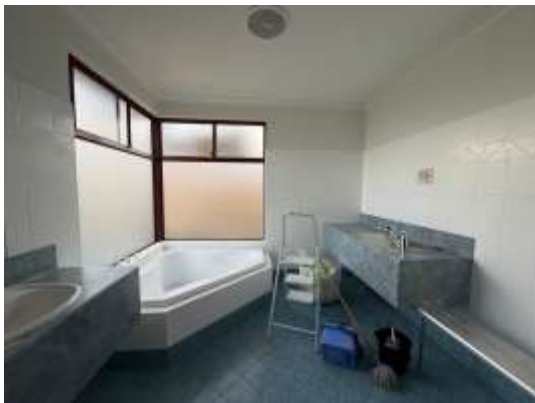
Amenities Family Bathroom Renovations underway
