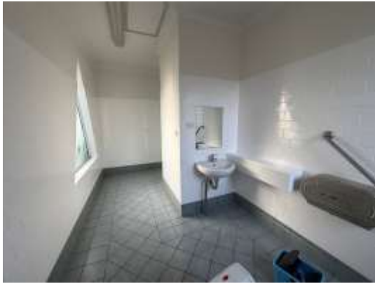
Amenities Accessible Bathroom Renovations underway
